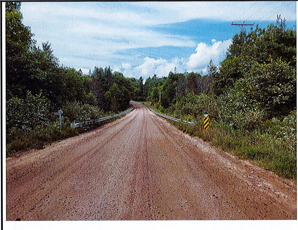
Photo 1 Structure from east approach
