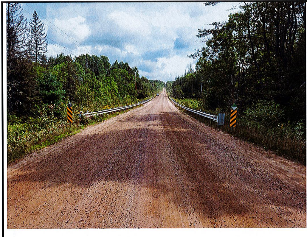
Photo 2 Structure from west approach
