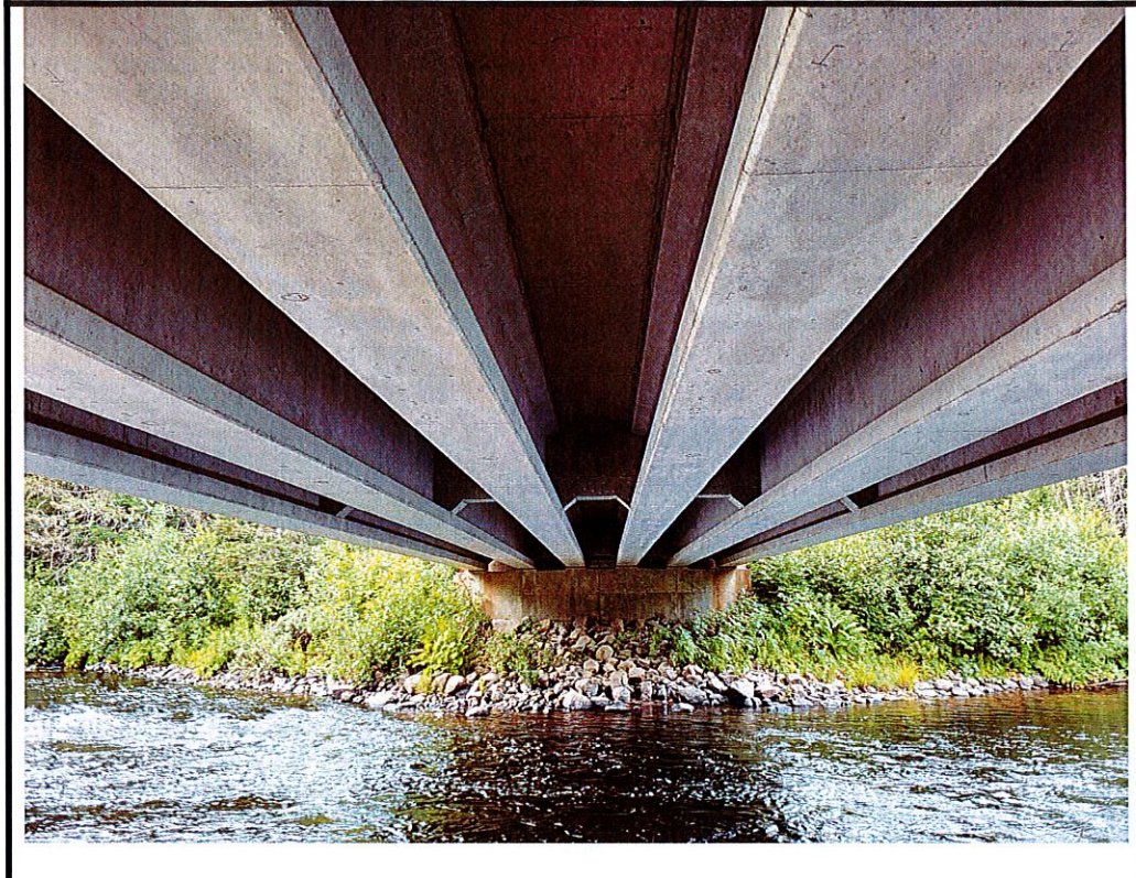
Photo 11 General view of girders and soffit
